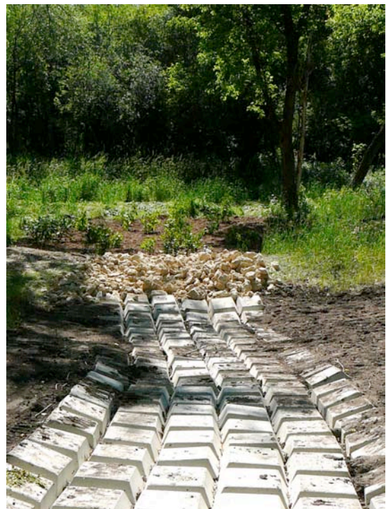
Ozark Avenue stormwater/rain garden project
