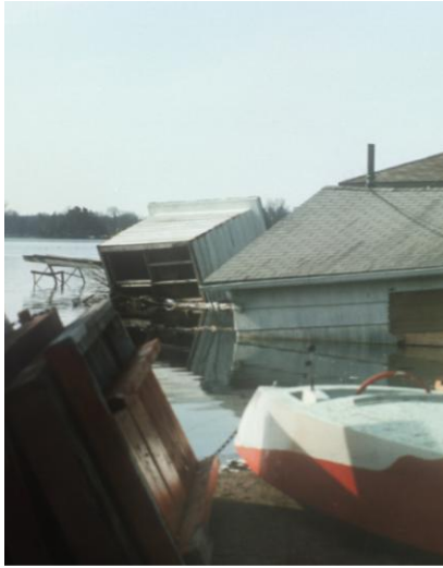
Big Marine Flooding prior to 1985 outlet project
